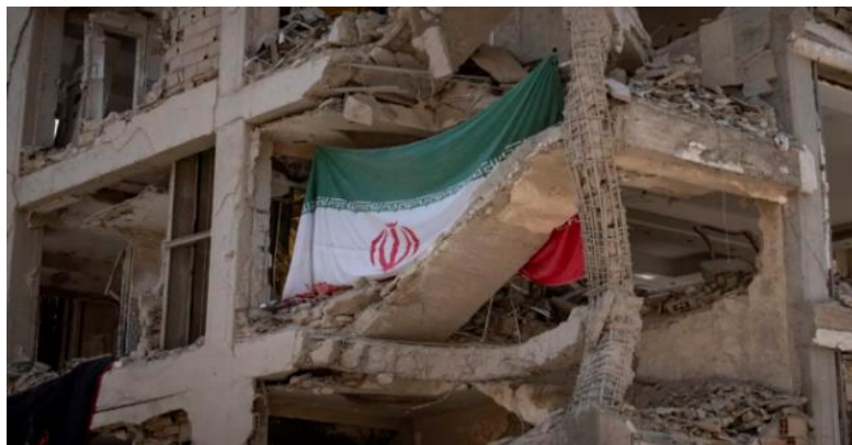
Iran building destroyed in US-Israel air attacks
